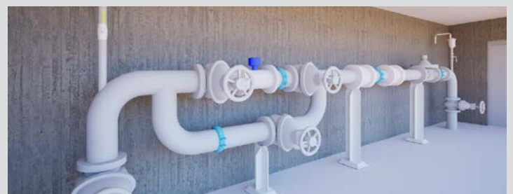
This rendering shows the types of valves and gateways housed within the turnout buildings that manage how water is sent from the main supply line into communities along the NGWSP.
